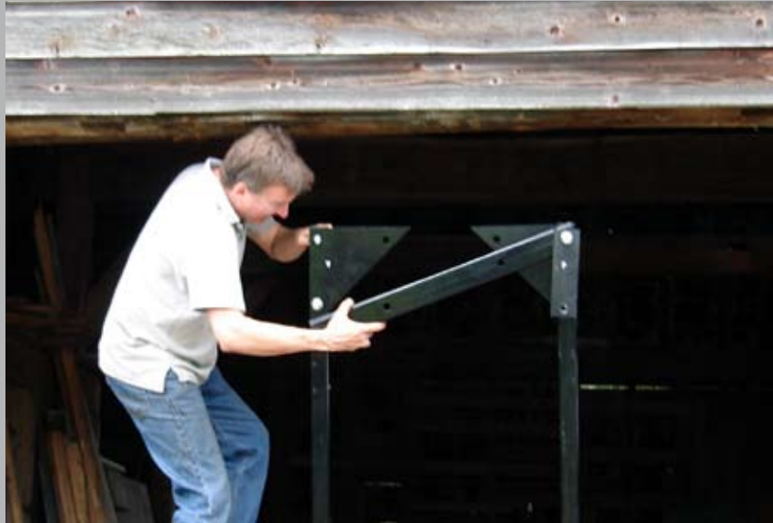
Steps 17-19 Installing Cross Bar Rear View
