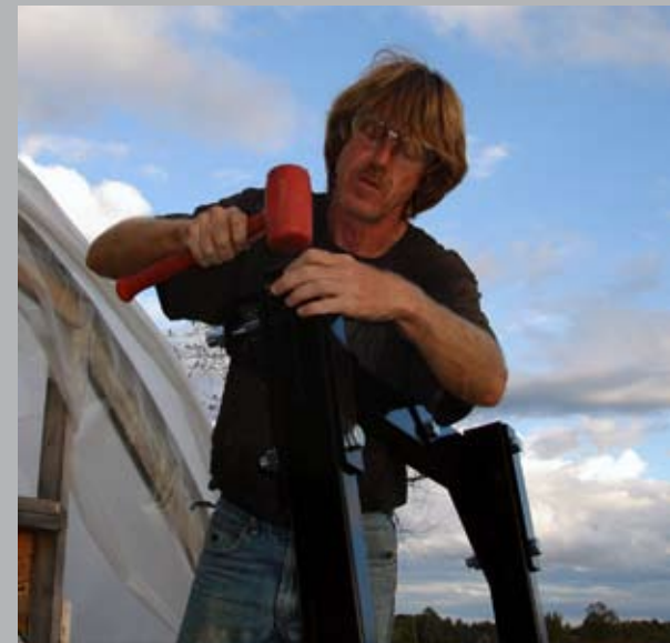
Final Step Install Plastic End Caps
